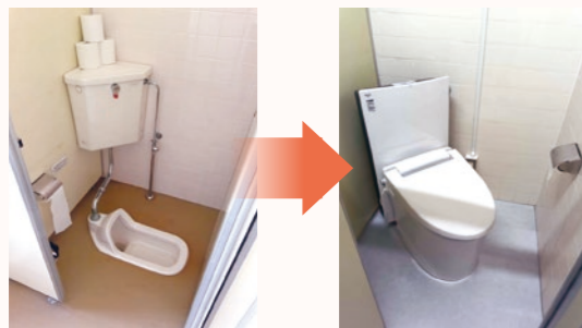
Before and after renovations
